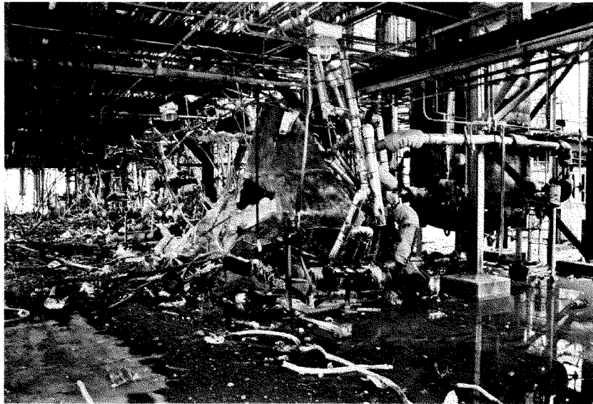
Figure 3: Equipment destruction along the trajectory of the residue treater vessel; the deformed shell of the vessel is visible at the center of the photograph.
