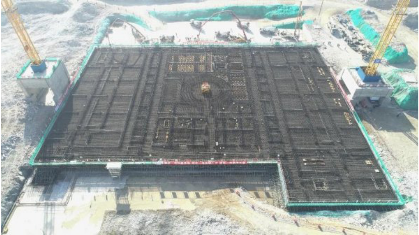
FIGURE 4. GROUND PHOTO OF THE SECOND CFR-600 UNIT IN EARLY STAGES OF CONSTRUCTION
