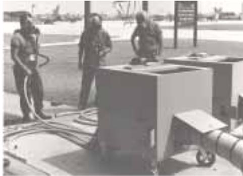
**6.3.1. Purpose.** The MICS provides cooling to alleviate heat stress to personnel performing moderate to high intensity work such as Integrated Combat Turn-arounds (ICTs) and some Base Recovery After Attack (BRAAT) functions while wearing chemical protective clothing.
