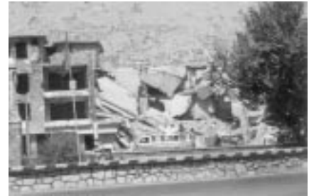
Demolished House in Kabul
