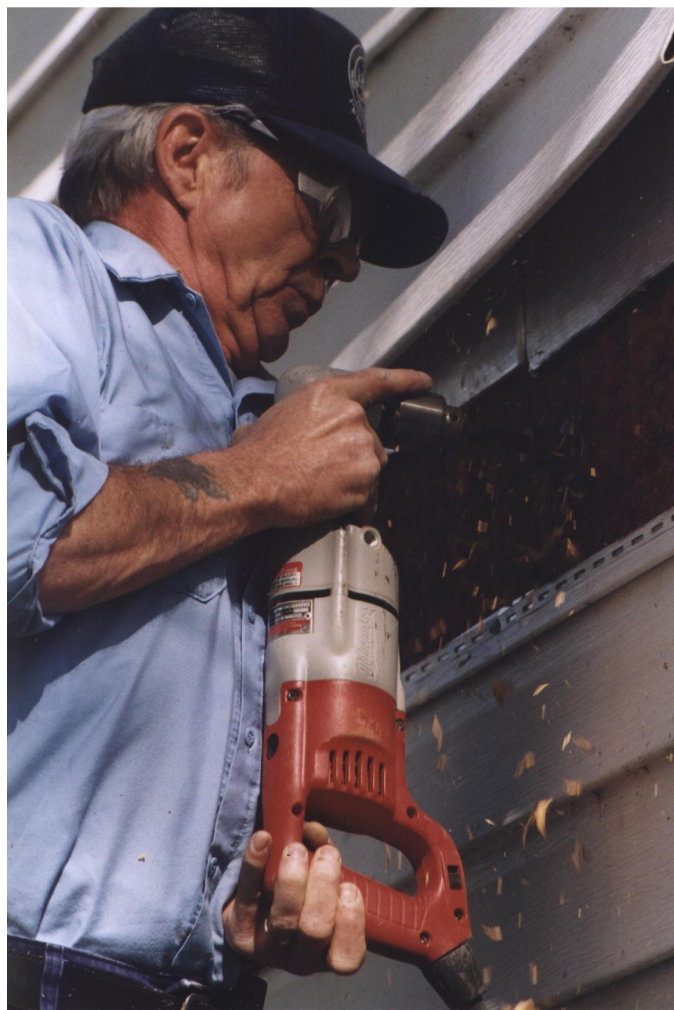
Preparing holes for sidewall insulation. 3
