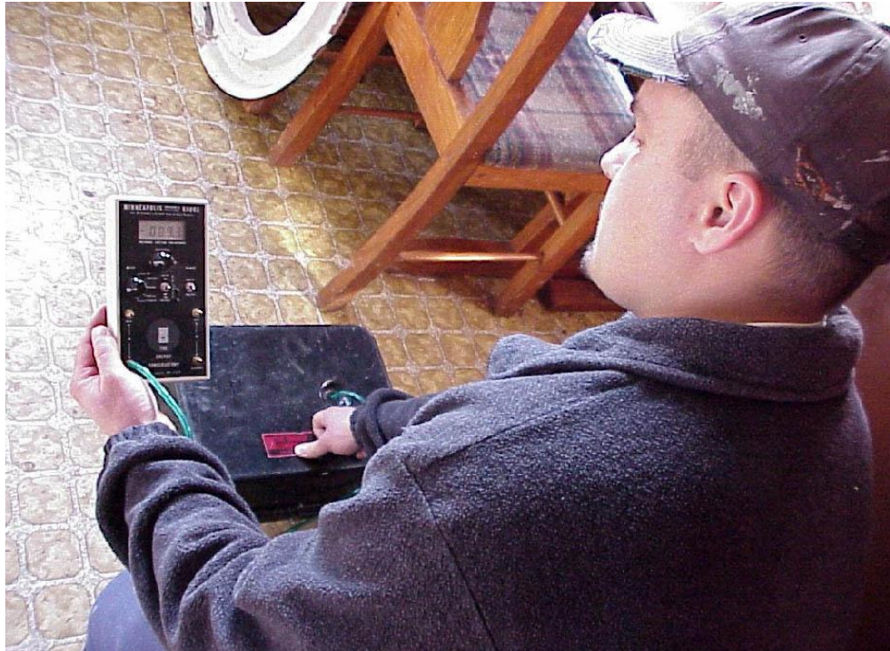
Diagnosing air pressure imbalances with manometer in West Virginia home. 10
