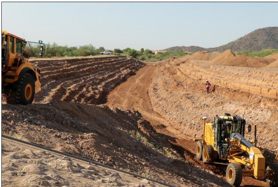
Figure 2. New River Dam Outlet Channel Repair Through P.L. 84-99 Rehabilitation Program
