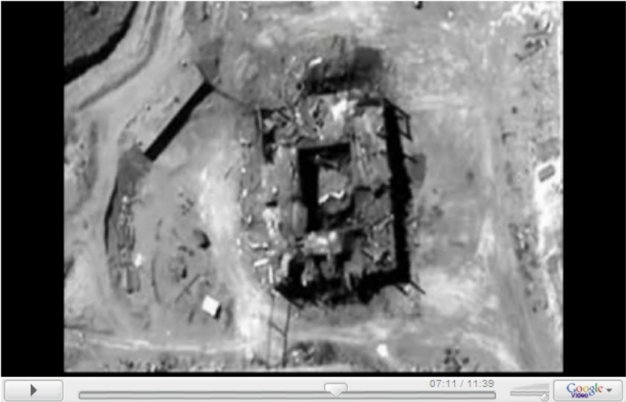
Reactor building after 6 September bombing and before 10 October demolition
