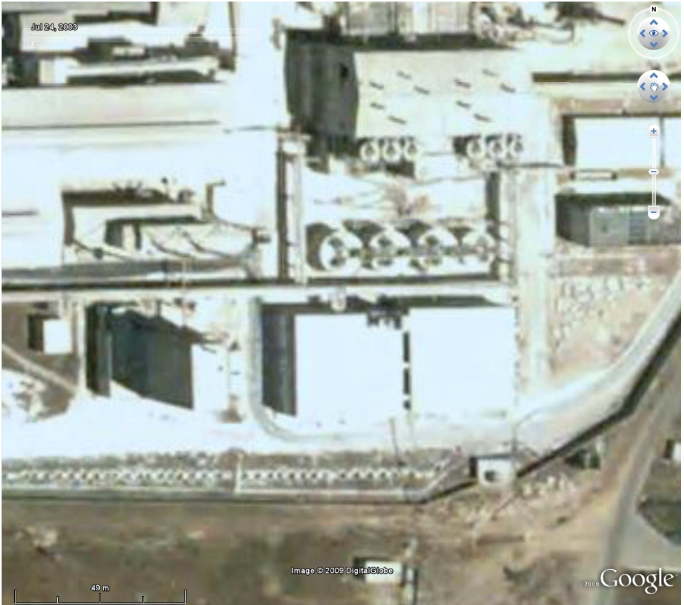
Closer view of separation facility
