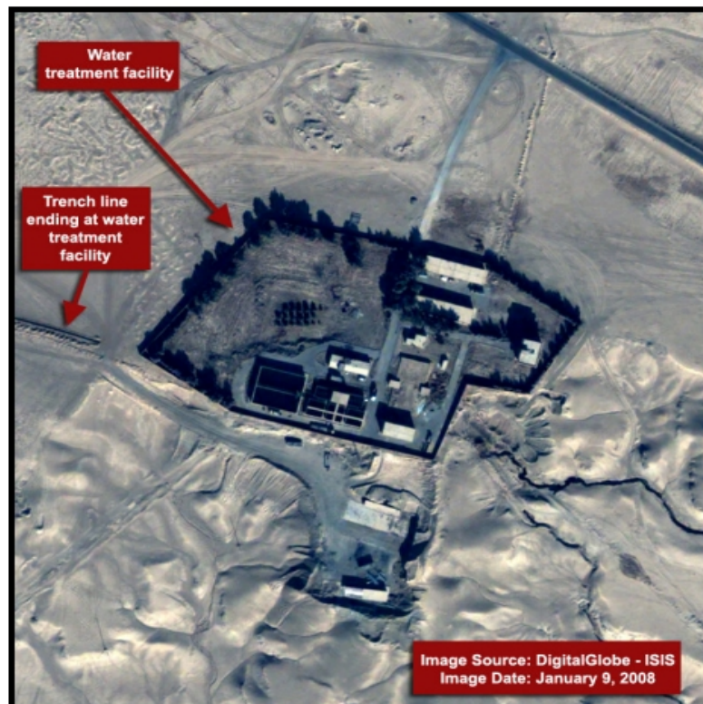
Figure 26. Image of water treatment facility after the reactor was destroyed.
