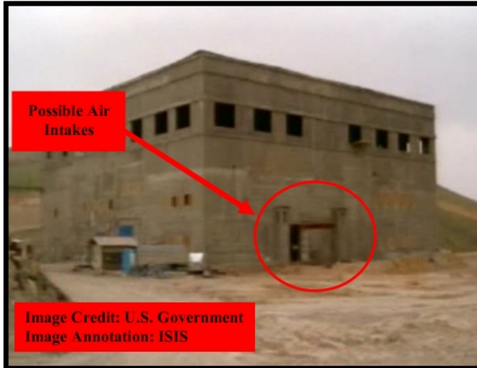
Figure 23. The air intakes for the Syrian reactor.
