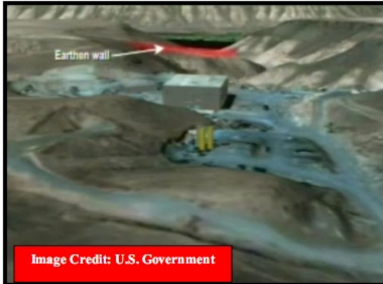
Figure 17. Location of an earthen wall on top of ridgeline.
