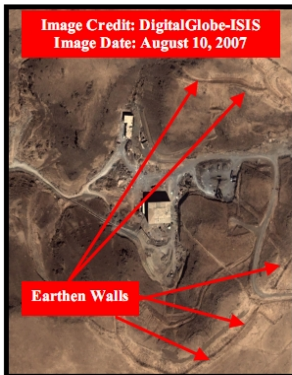
Figure 16. Syrian reactor site with earthen walls
