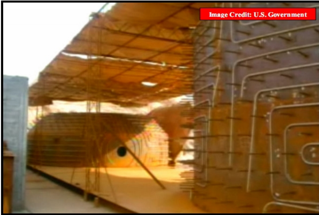
Figure 22. Syrian reactor vessel under tarps.
