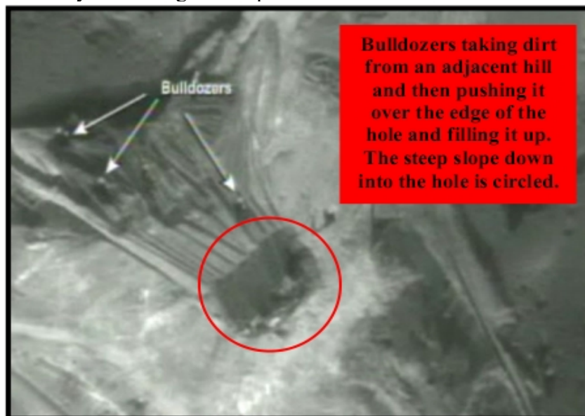
Figure 11. Bulldozers taking dirt from an adjacent hill and pushing it over the edge of the hole and filling it up.
