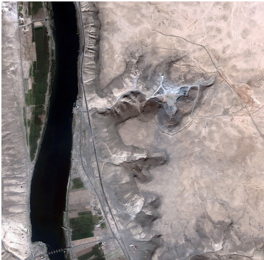
From above: A satellite image of the Syrian reactor site one month after it was bombed by Israeli forces in September 2007.
